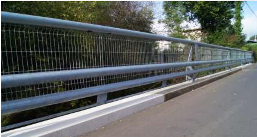
Fuse system allows the reuse of anchors after an impact
